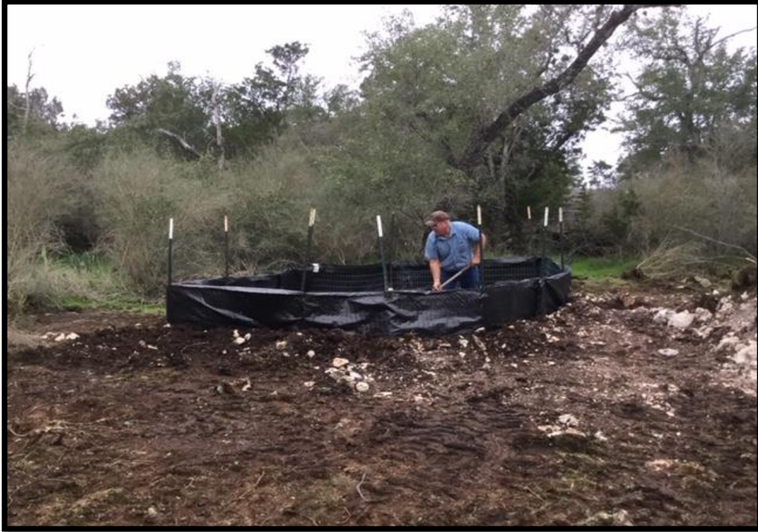
Photo 11. Silt-fencing placed around Features S-7/S-8 excavation site.
