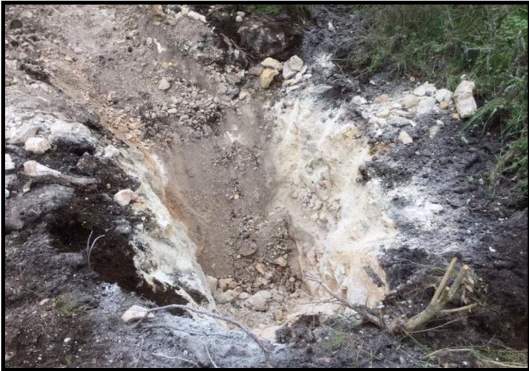
Photo 3. Excavation at Feature S-7 in progress through the resistant upper bedding unit of the Person Formation (Cyclic and Marine member).
